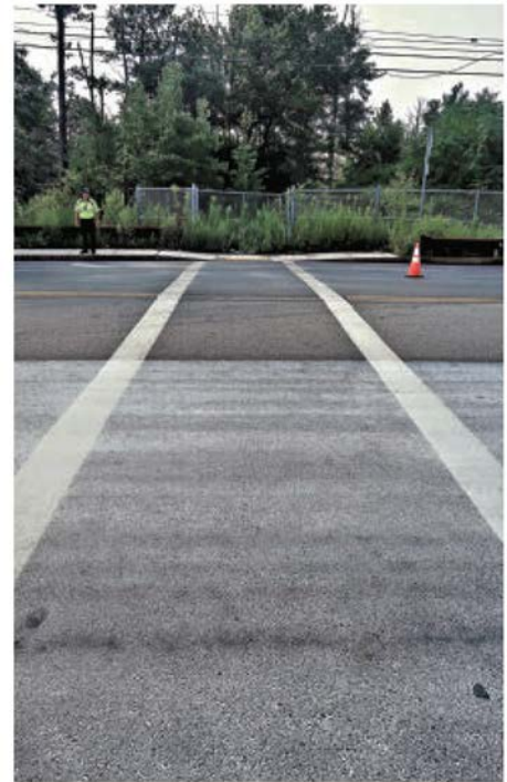
Delta Mist is applied in Bedford, Mass.
