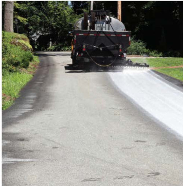
Bio-based rejuvenator is applied in Lexington, Mass.
