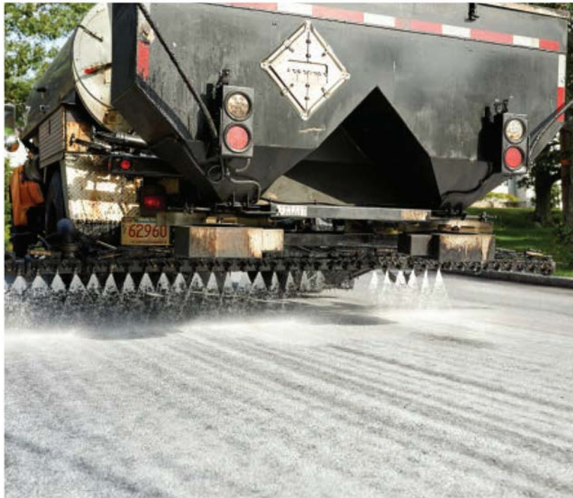
indus applies bio-based rejuvenator via distributor truck
