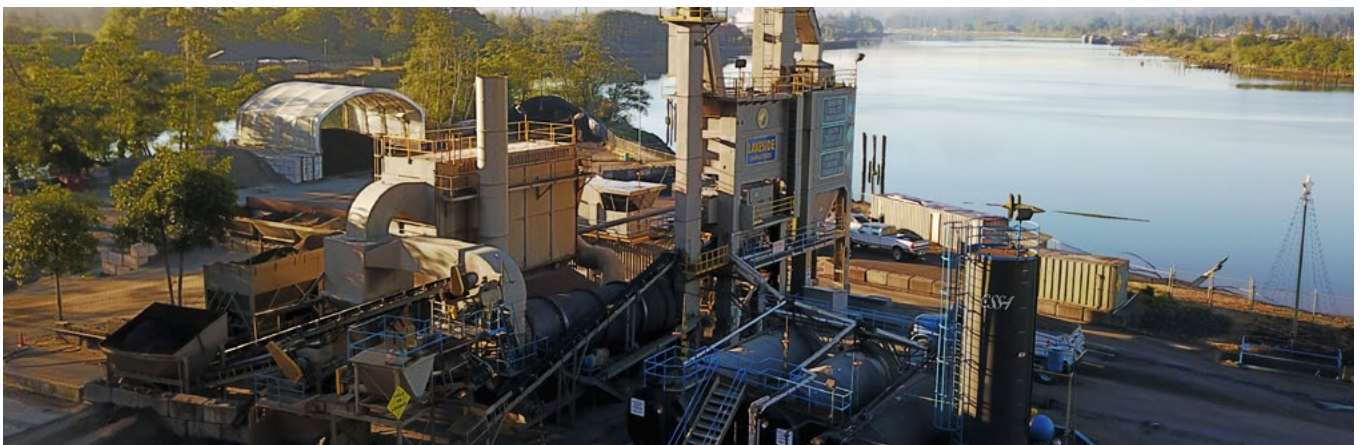
Aberdeen, WA, Asphalt Plant, courtesy Lakeside Industries
