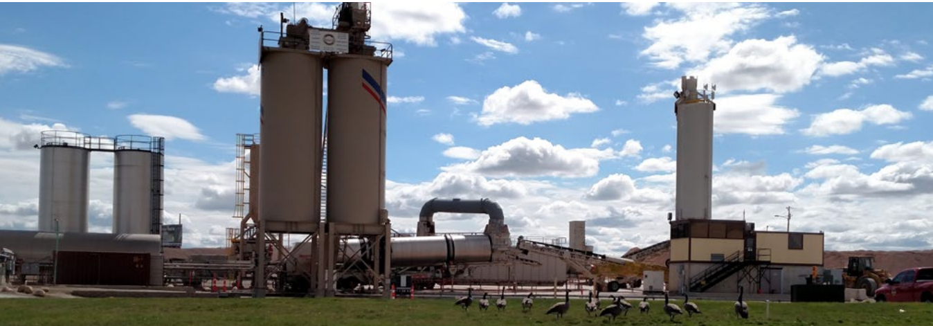
Gillette, WY, Asphalt Plant, courtesy Simon, a Colas Co.
