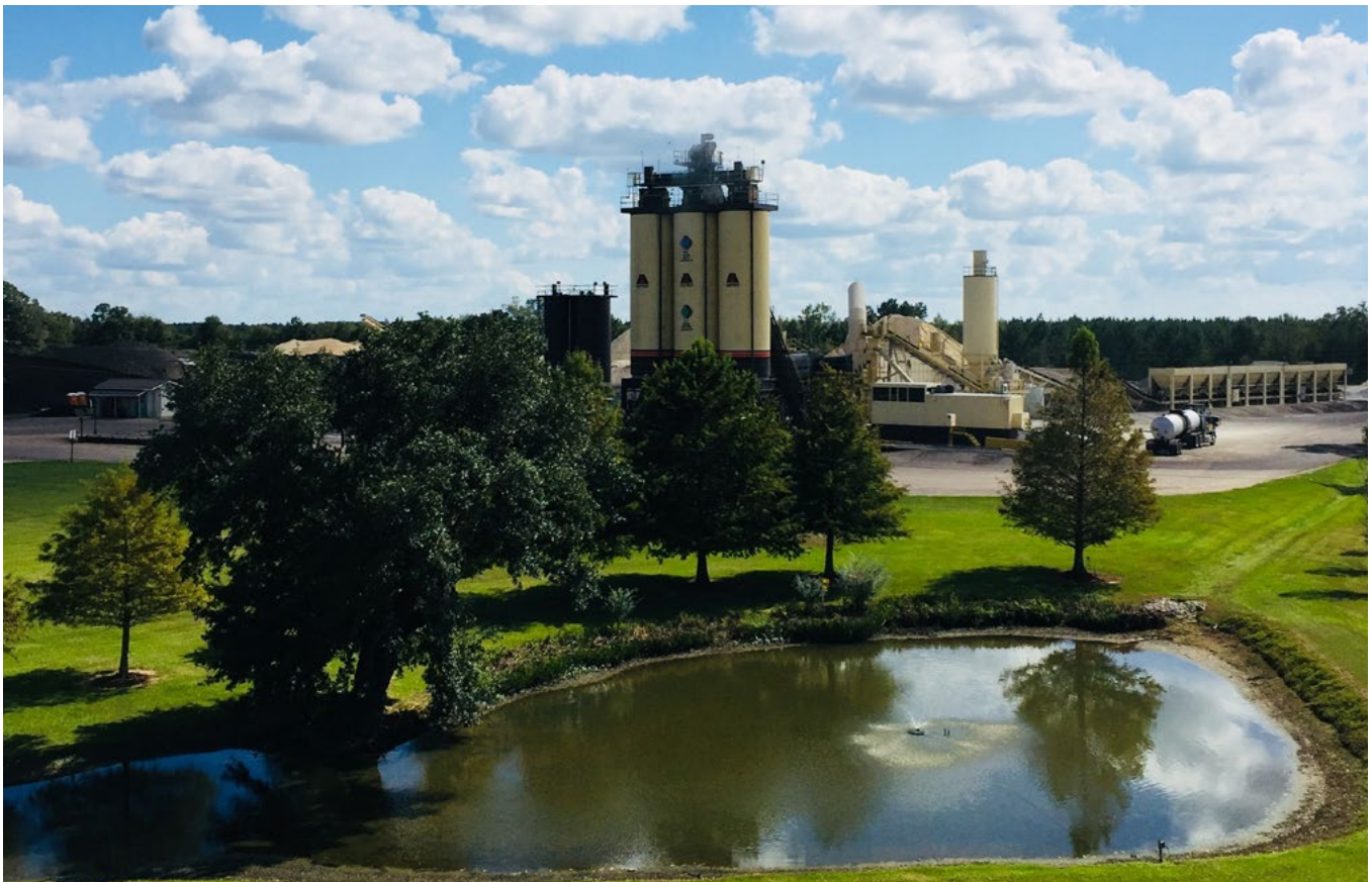
North Shore Asphalt Facility, courtesy Barriere Construction, A CRH Co.
