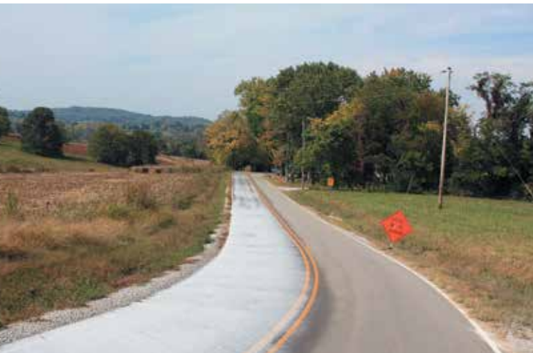
Plant-derived rejuvenator is white when sprayed, but turns clear as it dries. In this application, dry time was a little over an hour
