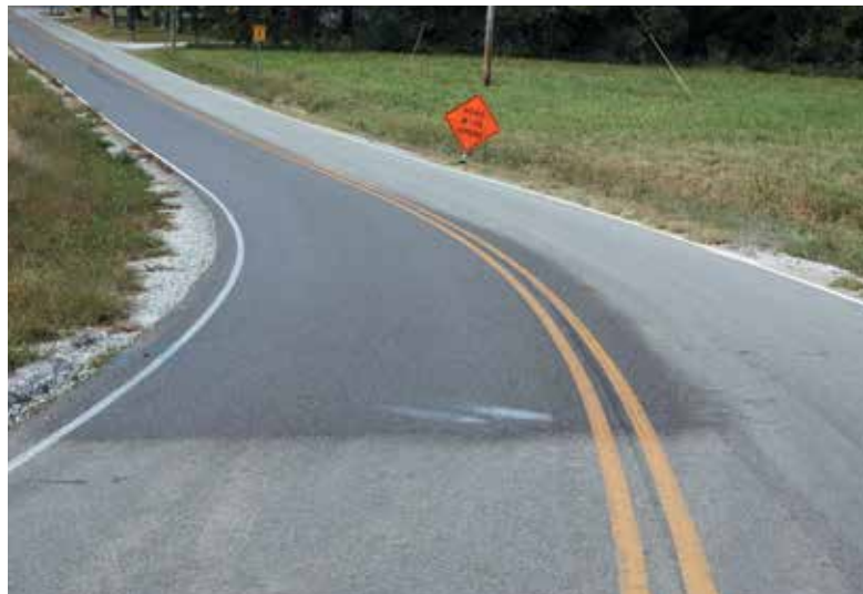
Dry application is transparent but leaves oxidized pavement a little darker
