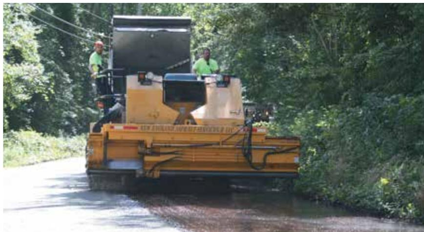
*New England Asphalt Services' Etnyre chip spreader drops chip seal aggregate as part of town's autumn asphalt pavement preservation program*
