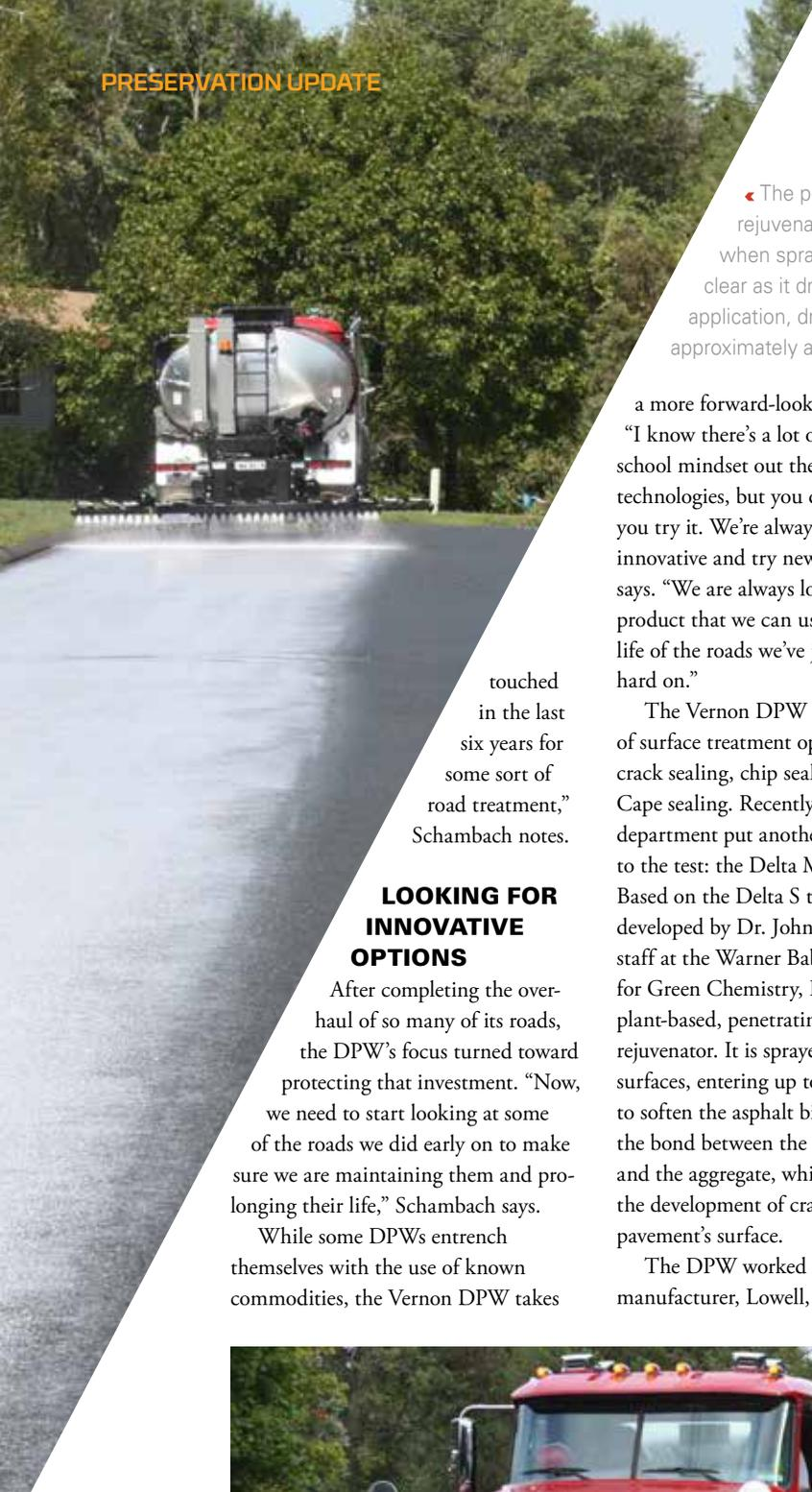
◀ The plant-based rejuvenator is white when sprayed, but turns clear as it dries. In this application, dry time was approximately an hour.
