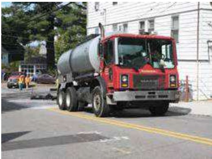
Riverside Asphalt sprayed the Delta Mist rejuvenator at a rate of 0.1 gallons per square yard.
