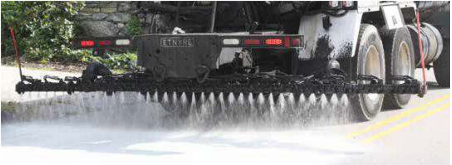
Riverside Asphalt sprayed the Delta Mist rejuvenator at a rate of 0.1 gallons per square yard.
