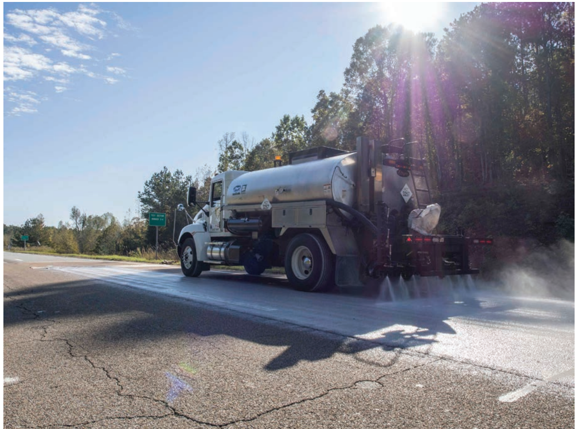
Delta Mist™ rejuvenator is applied to Section S3 of the NCAT Test Track.
