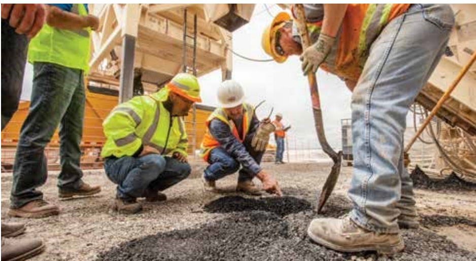
Delta S works by reversing oxidation of the asphalt cement (AC) through a carrier matrix. Bianchini explained that the plant-based carrier oil literally carries the remainder of the product into the existing asphalt binder where the other components of Delta S perform the chemistry of softening and reversing oxidation. Here Fujie Zhou (center, yellow hat) and William Still (white hat) discuss a sample of mix taken from the truck.
