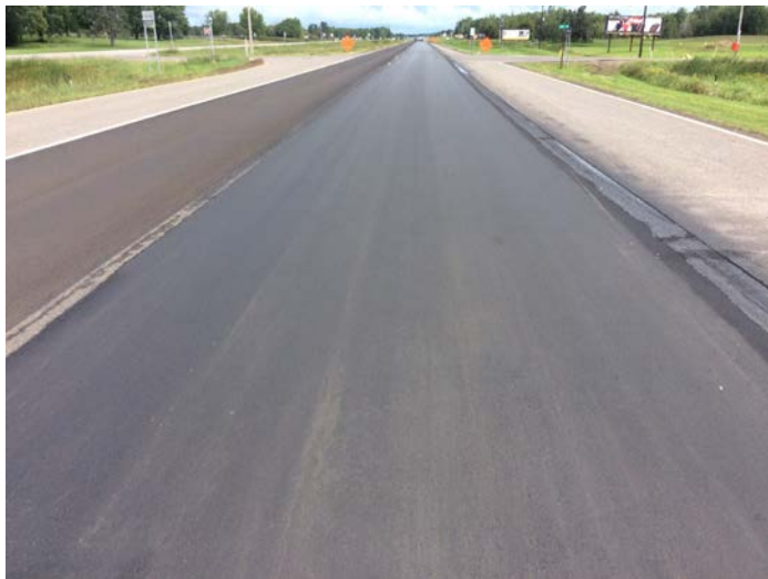
Cell 169022: As constructed in 2016.
