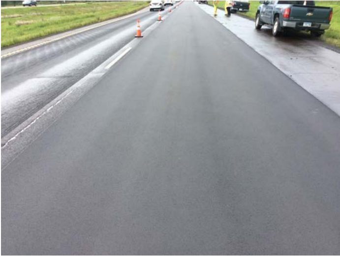
Cell 169026 as constructed in 2016.
