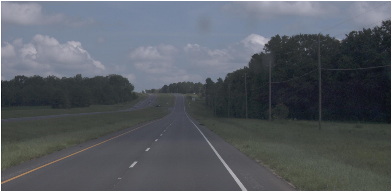
Figure 6. Post-Construction: Delta-S section.
