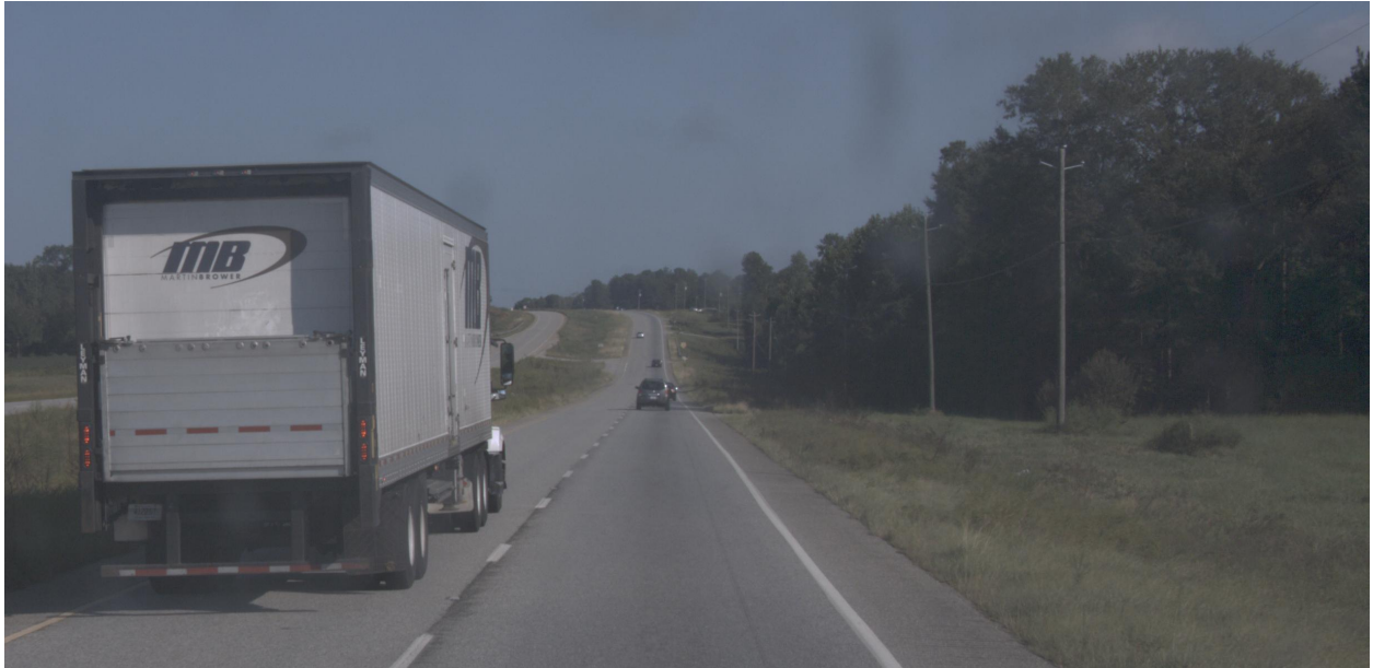
Figure 4. Pre-Construction: Delta-S section.
