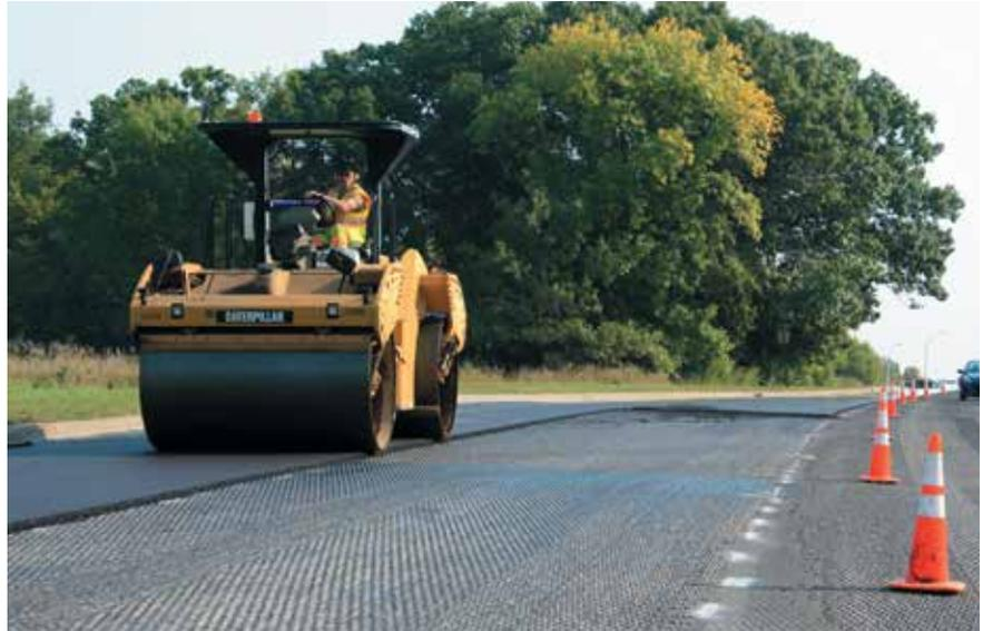
**The roller operator on the County Route 61 project has 35 years of experience and reported an easier time of rolling out marks from cross-traffic when working with the Delta S-dosed mat versus the control mat.**
