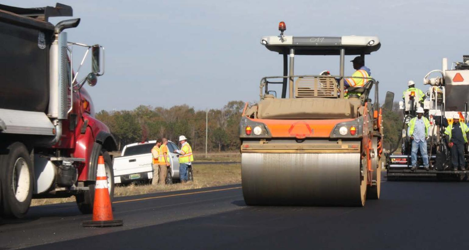
The Alabama Department of Transportation (ALDOT) is conducting an experiment on a four-lane highway involving an advanced, non-toxic asphalt rejuvenator in a pavement mix containing a high percentage of recycled asphalt pavement (RAP).
