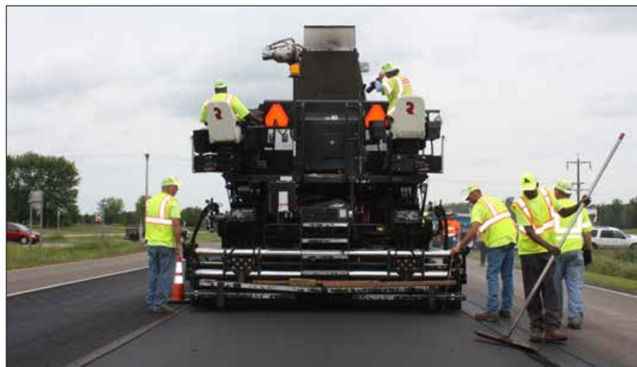
East Alabama Paving installs experimental asphalt mix in Minnesota using a Roadtec Spray Paver.
