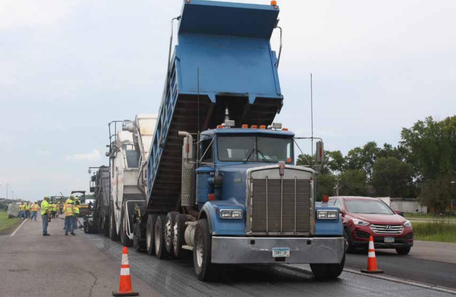
A truckload of hot mix asphalt containing RAP and asphalt rejuvenator is delivered to a Roadtec Material Transfer Vehicle for roadway pavement experiment in Minnesota.
