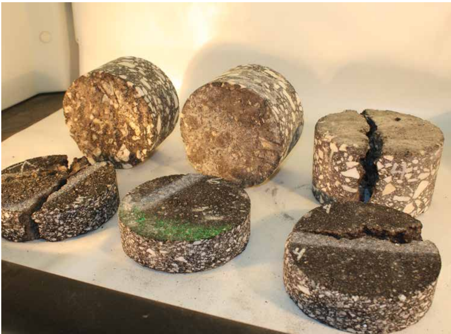
These core samples are from the original failed N7 pavement section.
