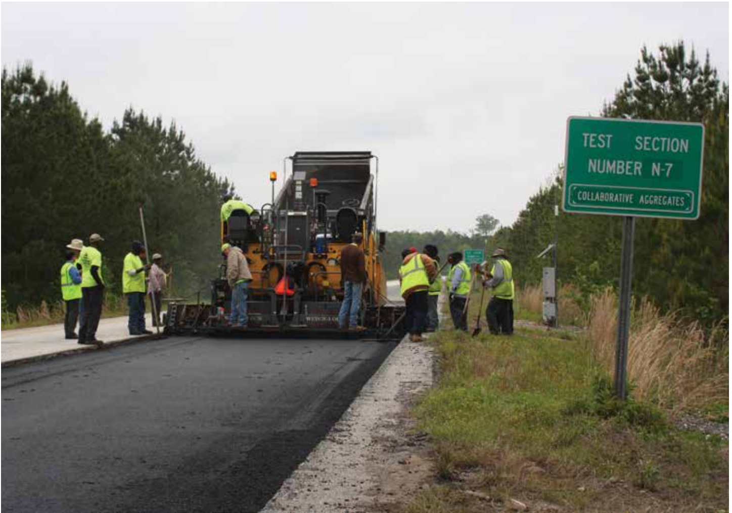
Here we see the crew installing the experimental asphalt pavement for section N7 on the NCAT test track in the summer of 2015. The 1.5-inch surface course included the Delta S rejuvenator.
