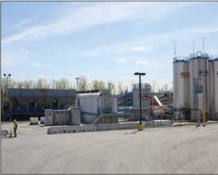
Delta S can be blended with liquid asphalt binder at the tank farm. Tilcon New Jersey adds the product to its mixes in-line during production.
